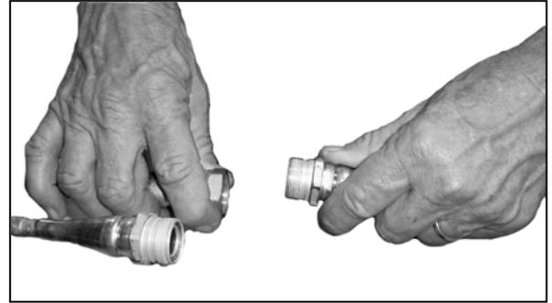
3. Once lines are uncoiled and run to the condensing unit and evaporator, line up the connectors and finger tighten the hex nut onto the male connector threads. **DO NOT CREATE ANY KINKS IN THE LINE.**
